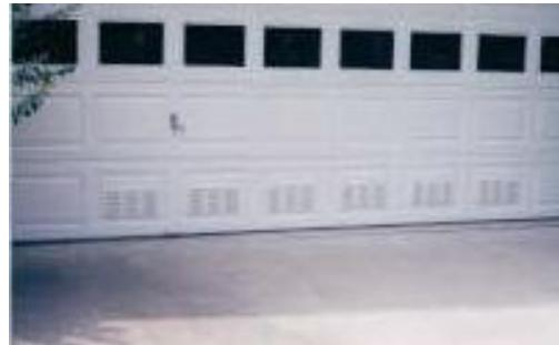
Several manufacturers have developed products that meet the flood venting requirements. Some of these products are certified to enable equalization of water pressure with smaller openings.
