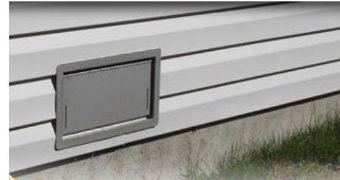
If the floor of the enclosure is below the Base Flood Elevation (100-year flood height indicated in the Flood Insurance Study and on the flood hazard map), then only those portions of openings that are below the Base Flood Elevation can be counted toward the required net open area.
